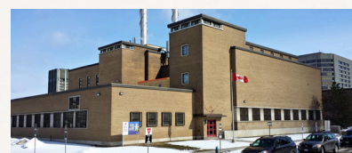
Tunney's Pasture Central Heating Plant by P199, via Wikimedia Commons. Licensed under CC BY-SA 4.0
